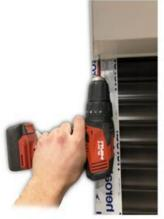
**(8.4)** Ensure that all opening gaps are sealed with silicone to avoid water penetration. For exterior applications, a rain drip cap is recommended. (Not provided.)
