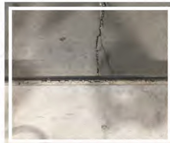
Cracked Concrete
