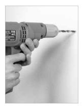
**4. Starter Hole.** Drill a starter hole the entire length of the drill bit (or to the tape marking  $2^{1}/_{2}$ -inches).
