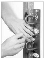
**8. Level.** Level the H2 unit and mark the middle and lower mounting holes.
