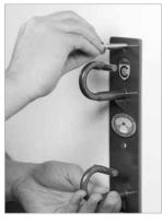
**6. Secure Lag Screw.** After the hole has been drilled into the stud, insert and tighten a lag screw until it is secure.
