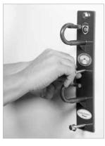
**10. Secure Lag Screws.** Tighten the lag screws until they are secure.
