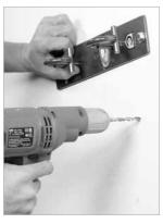
Drill Other Holes. Hold the H2 to the side and drill the other two mounting holes.
