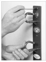
**2. Mark Hole.** Hold the unit in the desired position against the wall with the mounting hole directly on top of the centerline of the stud. Mark the top mounting hole.
