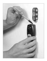
Studs. Locate a load-bearing wall stud using a stud finder. Mark the centerline (middle) of the stud.
