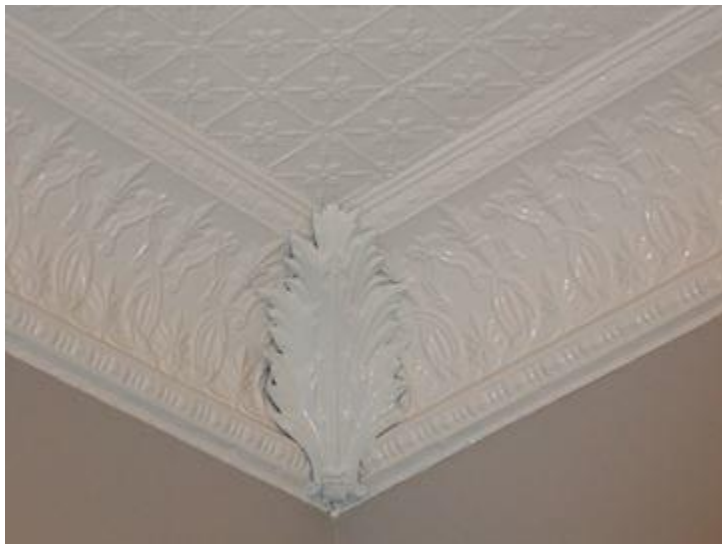
Elise Boyer had the tin ceiling of the Odd Fellows Hall restored and painted white. (Photo by Lisa Gillan)
