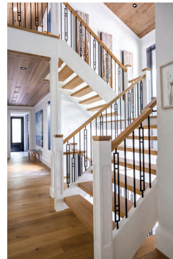
ABOVE: White oak, furnished by Ultra Carpet & Flooring, covers the hallway connecting the main living areas with the bedroom wing and stairway. LEFT: Deluxe Stair & Railing Ltd. used poplar, white oak and iron balusters to build the stairs connecting the cottage’s three levels. OPPOSITE: The homeowner designed the scissor trusses that support the high ceiling in the Muskoka room, where plenty of windows look out onto the surrounding forest and lake. Mac Masonry owner Mark Caruso built the stately floor-to-ceiling fireplace with cut and chiseled Indian granite from Northern Rock.
