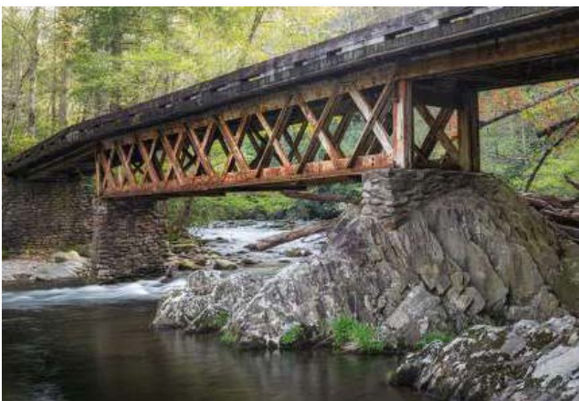
Title: Rusty Bridge SKU: POD-220702 https://northamericanart.com/products/rusty-bridge
