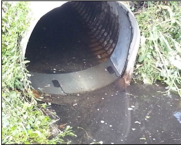
Figure 6 - AV sensors within surface water monitoring culver pipe (left), AV sensors installed within IDT discharge pipe (right)
