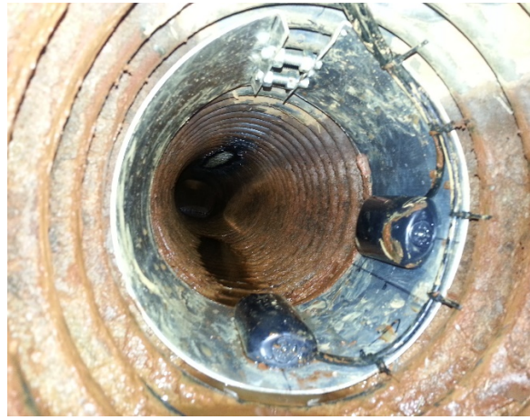
Figure 5 - Monitoring station at IDT field (left) and AV flow sensor within IDT discharge pipe (right)
