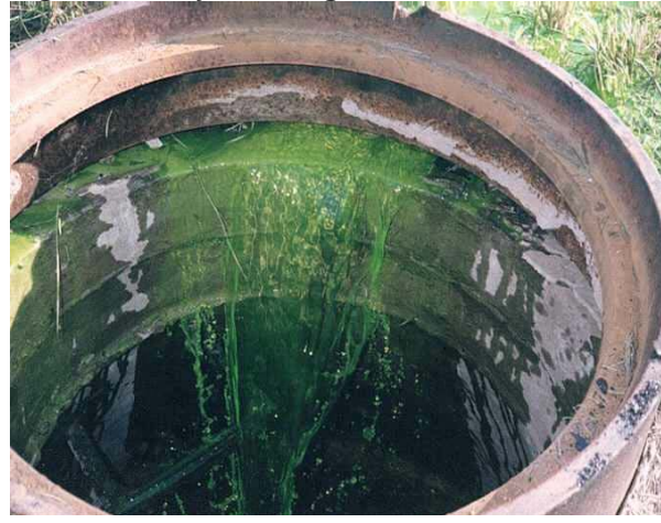
Figure 2.7. Dye Testing a Manhole
