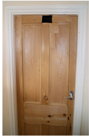
Rear of door
