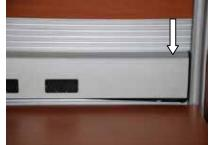
Place the raceway cover on top of the plastic cavaliers on each side of the panel.
