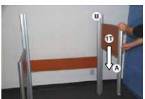
Slide half-panel 2 (48"W) in between the two 2-way posts B (57"H). Slide second panel 1T in between 2-way post B and second end-post A.
