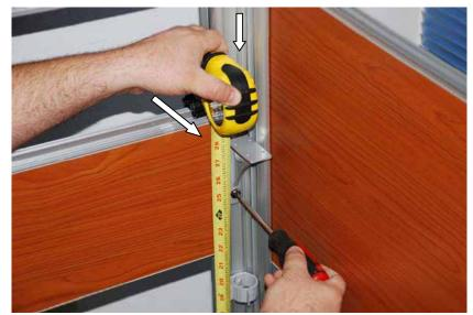
Adjust the brackets to the mark level (dot) showing on each post.
