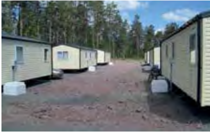
Temporary camp site with Sanicubic 1 systems
