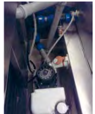
Pump installation behind oven
