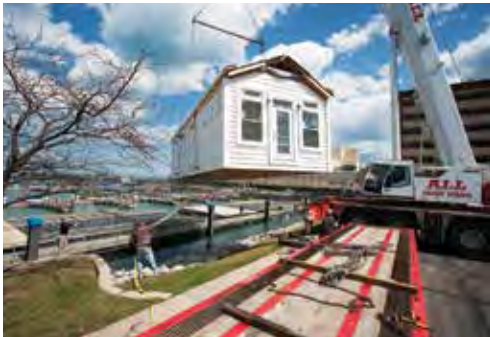
Crane used to place the bathhouse on to floats
