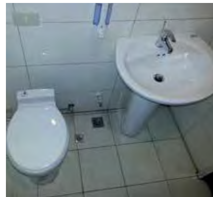
Sink connected to Sanicompact macerating toilet and pump system.
