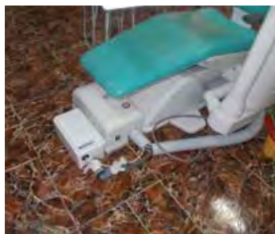
Dental chair equipped with Sanishower drain pumps
