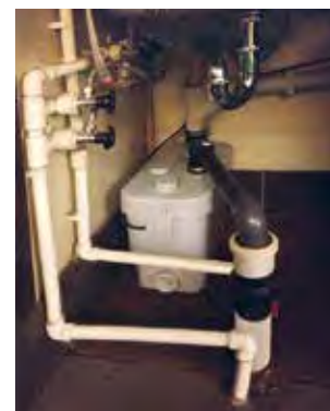
Sanivite installed underneath the counter sink
