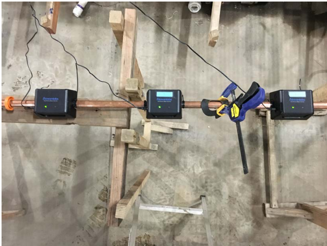
Figure 2. Streamlabs copper pipe installation
