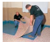
Cellular polyurethane layer
