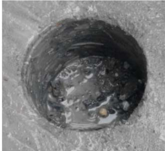
Figure 5. drill a hole
