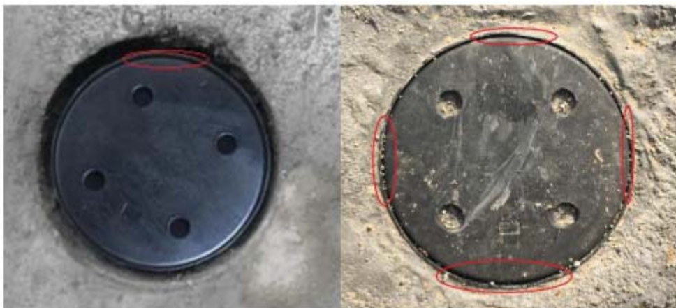
Figure 6. the spiral slit is marked in red circle
