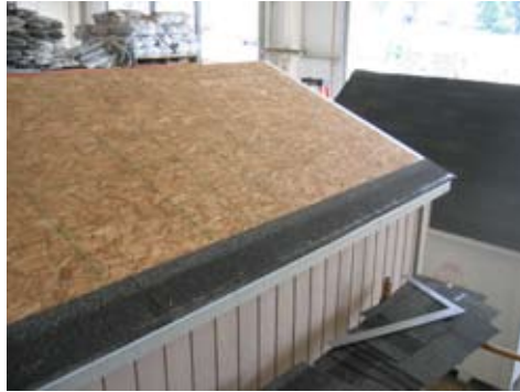
This shows more shingle installation.
