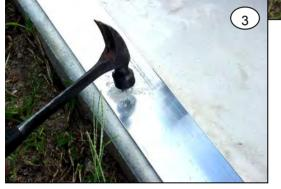
Insert the 1/4" drive pins into the holes and anchor the ABA to the concrete using a hammer as shown in **photo 3**.
