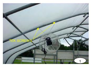
USE THE CHAINS PROVIDED TO ATTACH HAF FANS DIRECTLY TO THE BOW ASSRMBLY OR TRUSS CHORD. USING TEK SCREWS,SCREW THE CHAINS DIRECTLY TO THE SIDE OF THE BOW ASSEMBLY AS ILLUSTRATED IN PHOTOS 1 & 2.
