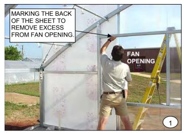
Begin with the first sheet flush with the outside corner. Be sure the sheet is vertically level and in its proper location. Trace out any door, fan or shutter openings on the backside of the sheet and remove the excess using a skill saw. (See photos 1& 2)
