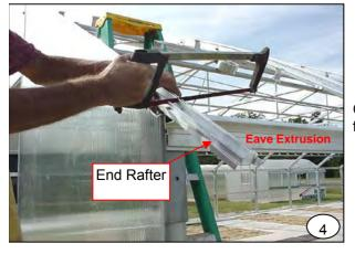
Cut off the excess, making sure that the end rafter extrusion stops flush with the edge of the eave extrusion. (See photo #4)
