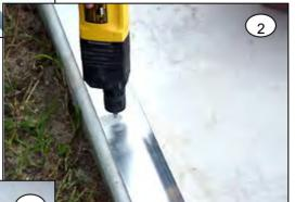
Next use a 1/4" masonry to drill the holes into the concrete footer approximately 3" deep. (*Photo 2*)
