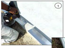
Using a metal cut bit, drill a 5/16" hole approximately every 18" apart down the length of the ABA. (*Photo 1*)
