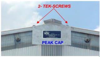
Finish off the end walls by capping each gable end peak, using a peak cap. Allow the 1-1/2" flange of the peak cap to slide between the end rafter extrusion and the snap cap until the peak cap is lying flush against the end wall. Center the peck cap and insert two #12 x 2" washer tekscrews through the aluminum cap, the peak cap and into the end rafter extrusion. (See the above photo & Fig. J)
