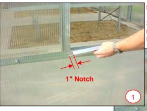
Measure the bottom of the opening and notch the 1"  $\times$  1" angle leaving 1" extending beyond the opening on both ends. (See photo 1) Slide the angle into the opening and attach it from the outside using the # 12  $\times$  1" tek-screws provided as shown in photos 2 & 3. Repeat these steps for the top of the opening.
