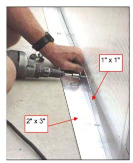
Identify and attach the 1"x 1" aluminum angle. This 1" aluminum angle lies over the 2" x 3" Aluminum Base Angle (ABA) and against the P.C.S.S. at the base of the structure.
