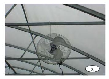
THE HANGING BRACKETS CAN ALSO BE USED TO ATTACH THE HAF FANS TO A TRUSS CHORD WHETHER IT BE SQUARE, RECTANGLE, OR ROUND TUBING AS SHOWN IN PHOTO 3.
