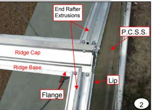
Starting at the top, lay the end rafter extrusion over the flange of the ridge base extrusion making sure that the lip is turned down lapping the P.C.S.S. endwall covering. Butt the end rafter extrusion up to ridge base extrusion and insert two screws into the end rafter extrusion, through the flange of the ridge base extrusion as shown in **photo #2.** (Also see Fig. F)
