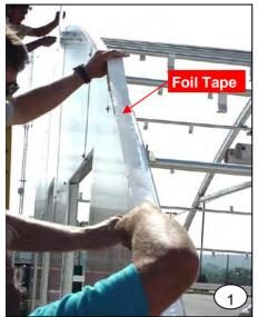
Apply foil tape to the top of the end rafter, allowing it to over-lap the top edge of the P.C.S.S. endwall covering. This prevents moisture, caused by condensation from collecting between the two layers of the P.C.S.S. covering. (See photo #1)
