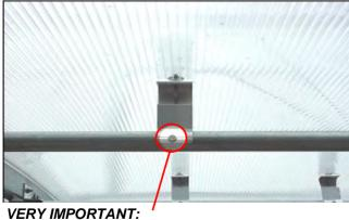
Once all the P.C.S.S. roof panels have been installed, you must insert a tek-screw through each of the P.C.S.S. support brackets into the purlins. Failure to do so, could result in structure failure in severe weather conditions.
