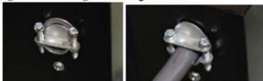
Figure 11: Installing cable fitting to heater
