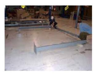
Step 5: Connect the main beam (the one without angle bar) into the posts and lock it on the second lock. Then put both posts up. Please refer to below picture.
