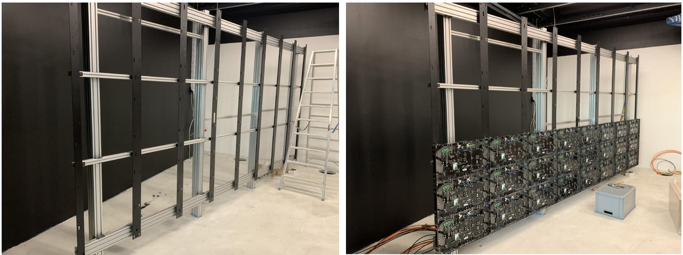
The entire project process from start to finish was reliably and professionally supervised by the Peerless-AV team. The dvLED video wall was the critical part. Peerless-AV designed and manufactured and delivered a Kitted+ Series dvLED Mounting Solution consisting of bolt down substructure and mounting system with dedicated adaptors to support Unilumin Upanel II 1.2mm pixel pitch, front maintenance, cable-free cabinets in an 8x7 wall configuration, measuring 4.8 m (W) x 2.4m (H).
