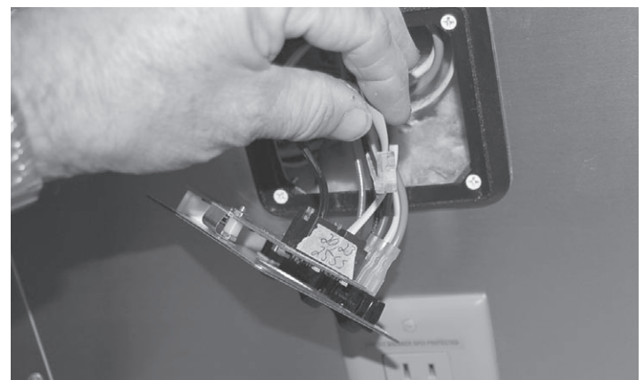
Fig. 5. The leads from the tanks are plugged into the back of the monitor's faceplate with telephone-type RJ-11 connectors. Remove only the ones you do NOT want to calibrate. (The leads are colored and the lead sockets are labeled so you will know where to plug them when you reconnect the leads to the faceplate.)
