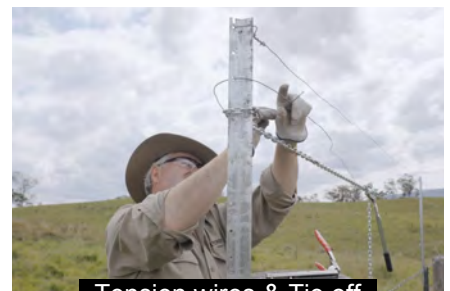
Tension wires & Tie off
