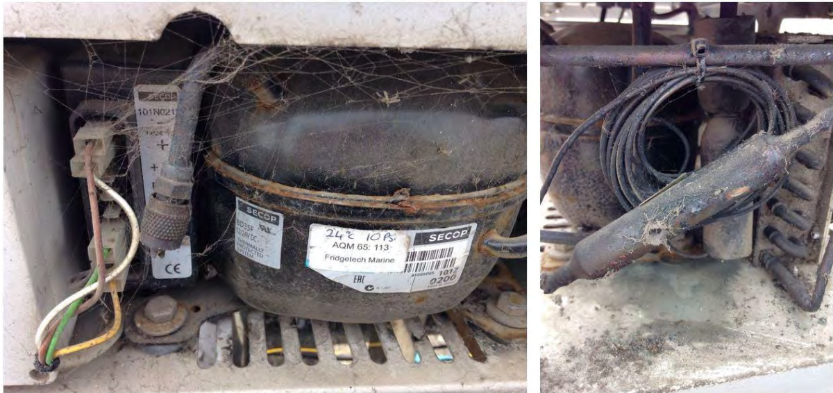
Figure 4-29 Dirt and debris can accumulate within the TMS cassette leading to reduced efficiency of the thermal management system.
