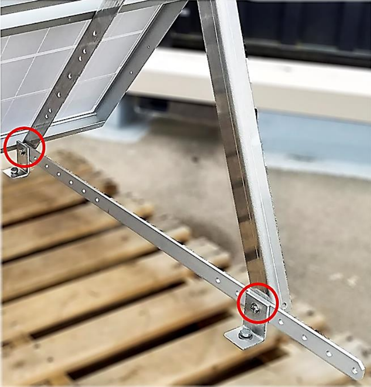
Figure 36: Fasten Two Flat Bar Pieces
