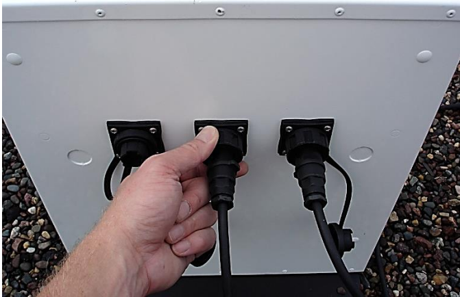
Figure 38: Connect Solar Cells to Battery Enclosure Box
