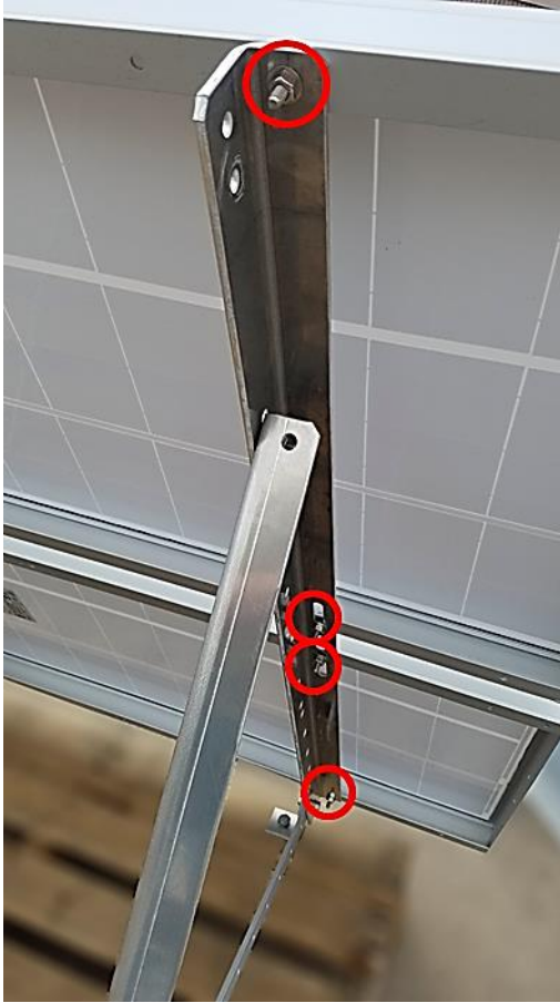
Figure 34: Assemble the Solar Cells on the Mounting Frame
