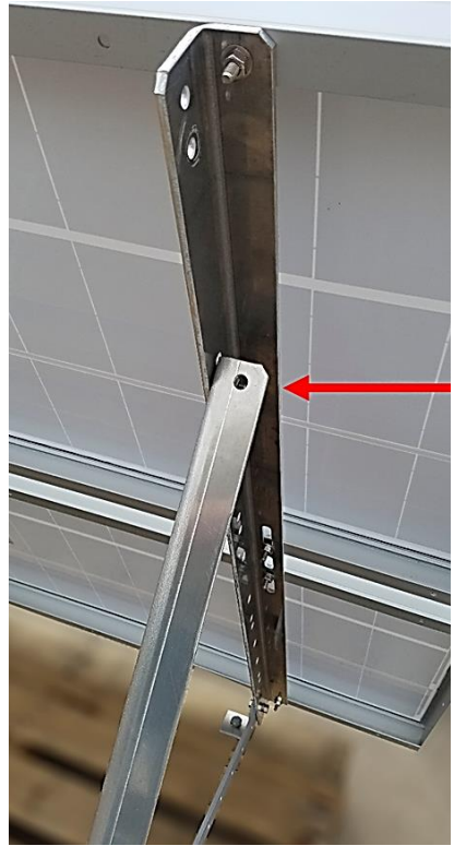
Figure 35: Attach Shorter Structural Angles
