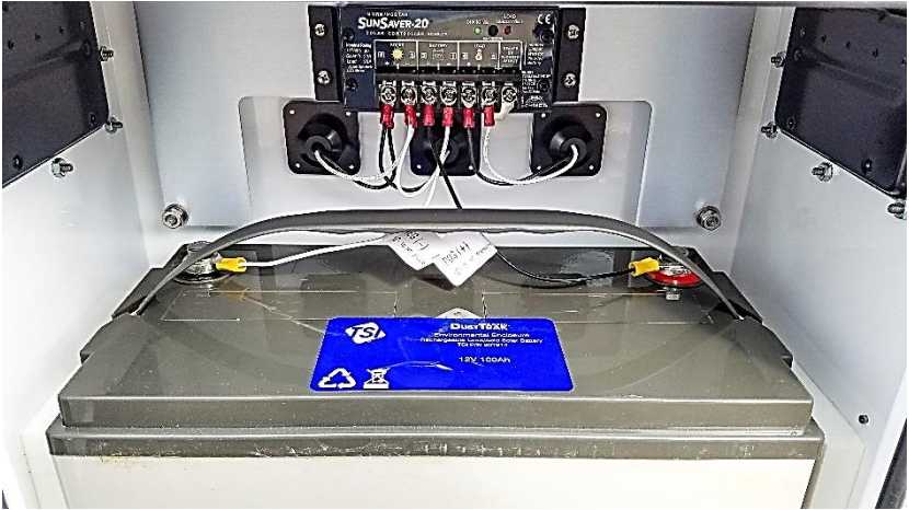
Figure 27: Install the Solar Battery and Connect to Controller
