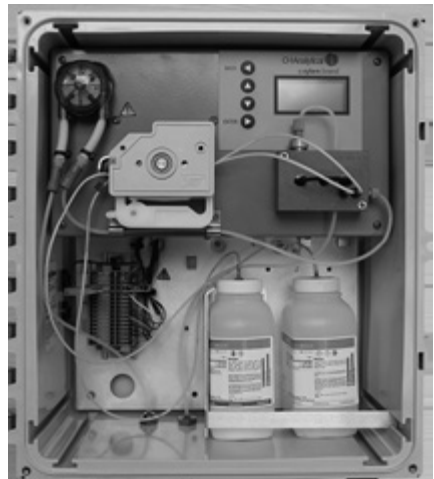
Figure 6: Completed pump tube installation
