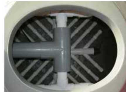
Lateral under drain system
