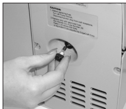
Figure 10. Replacing the fuse located underneath motor housing.
