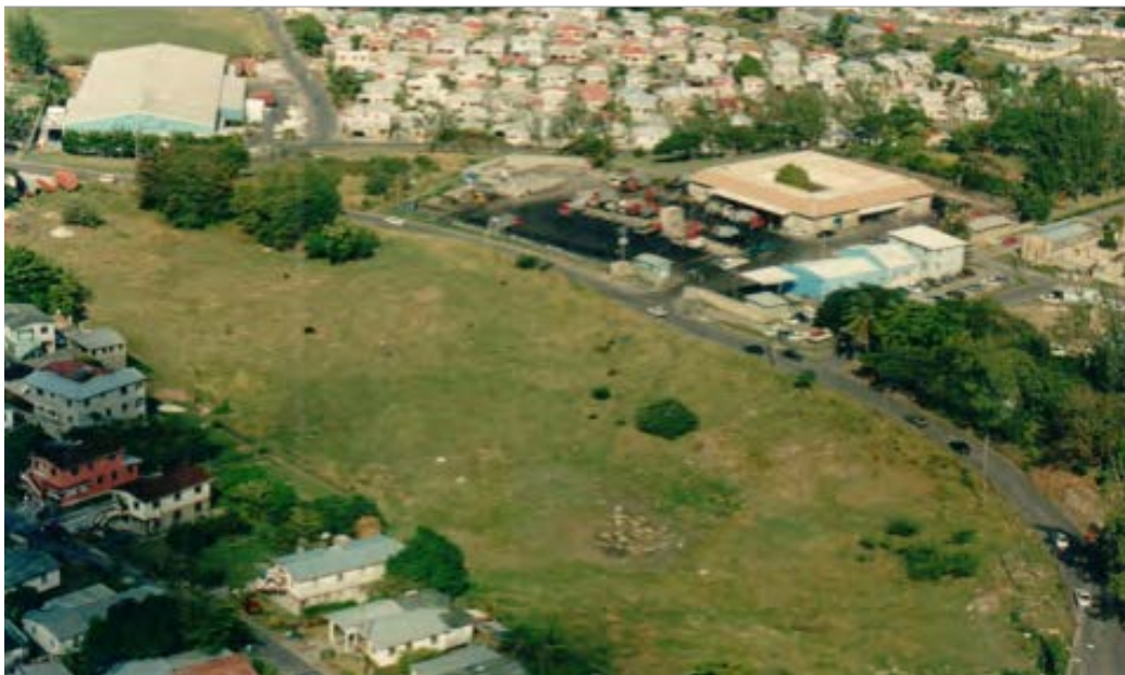
Adjacent lot opposite Sanitation Service Authority base, earmarked for the development of Wildey B - warehouse, retail store and corporate offices.
