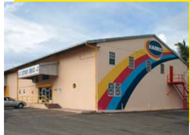
Bois D'OrangePaints; Under Construction (top), Completed (bottom)
