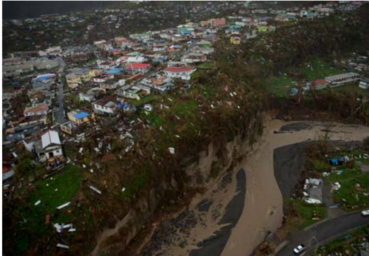
Aerial view of the devastation in Roseau, Dominica on 28 September 2017 (Photo by Jose Jimenez, Getty Images)
