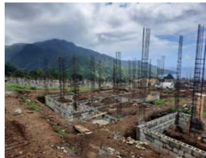
Foundations underway at Grand Bay (2022)
