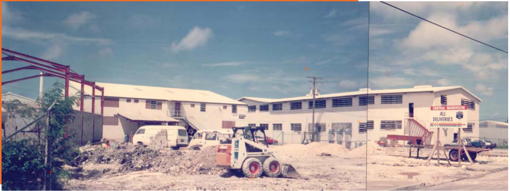
Building of Wildey factory in progress
