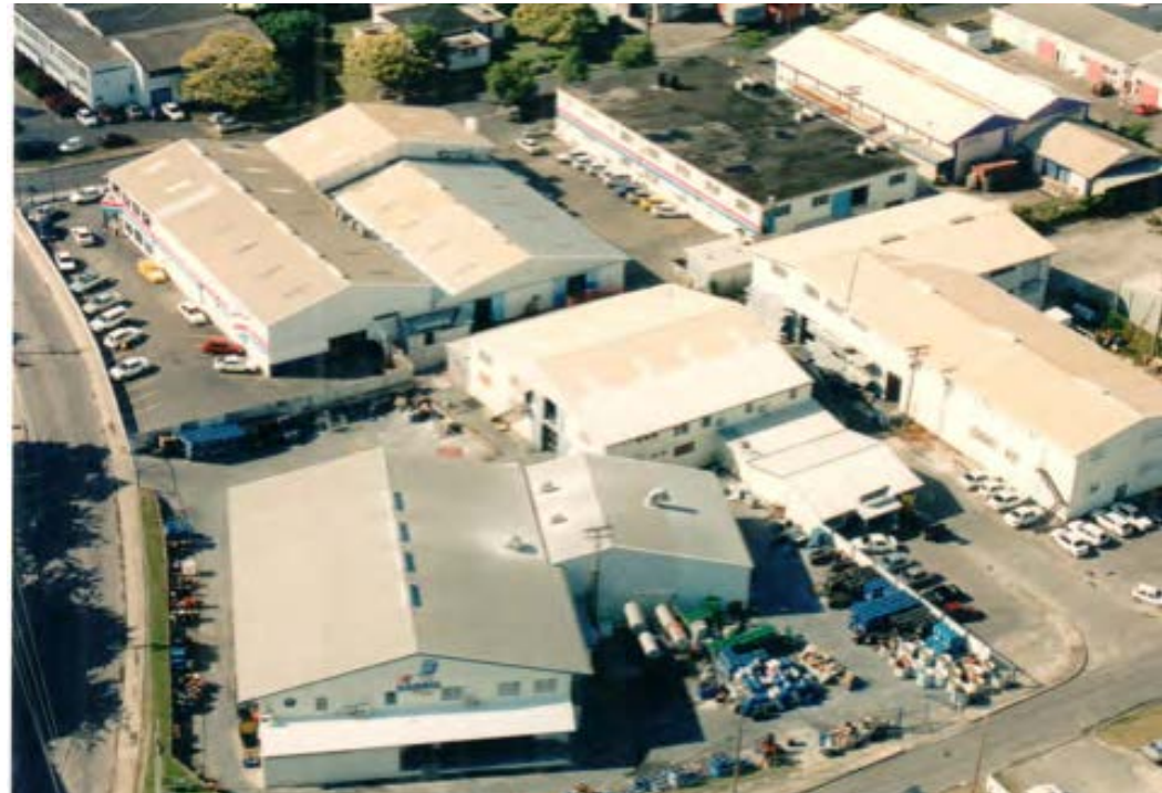
Aerial view of original Harris factory lot in Wildey (Wildey A).
