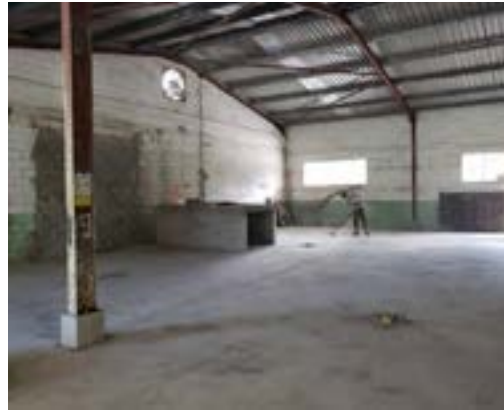
Cleared and cleaned
