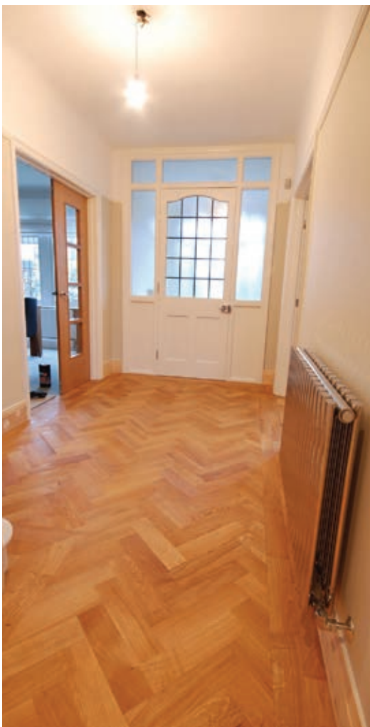
White Oiled Maple 37.5 degree DIAGRID parquet pattern with bevels for easier installation
