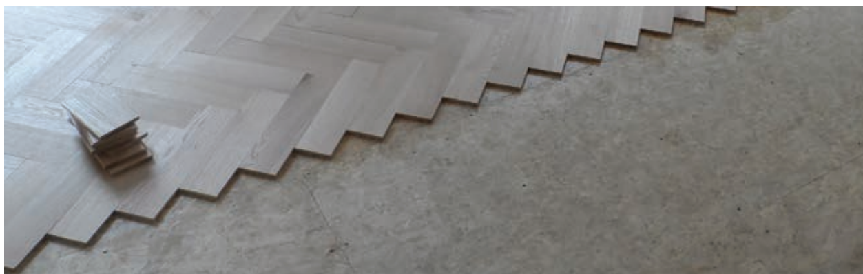
Fitting our overlay parquet blocks
