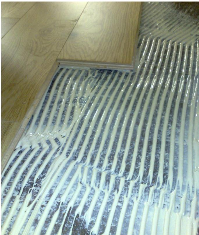
The image on the left is the correct application of the SW890 adhesive.
