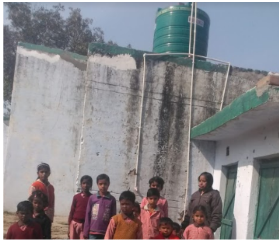
Figure 2: Freshwater connection with an overhead syntax tank.
