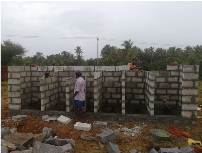
Bio-toilets under construction
