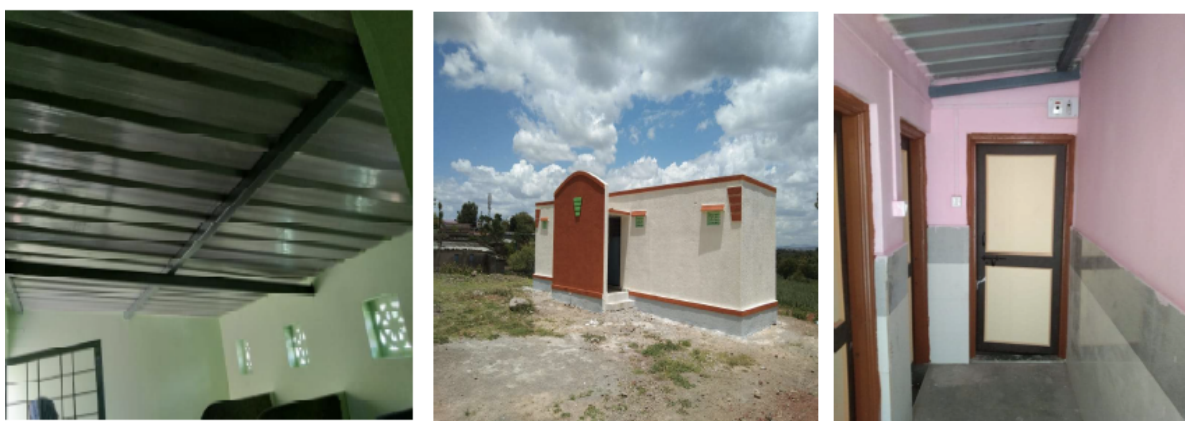
Figure 1: Completed sewa toilet units @ Mahura madhyamik vidyalay, Pune - Maharashtra
