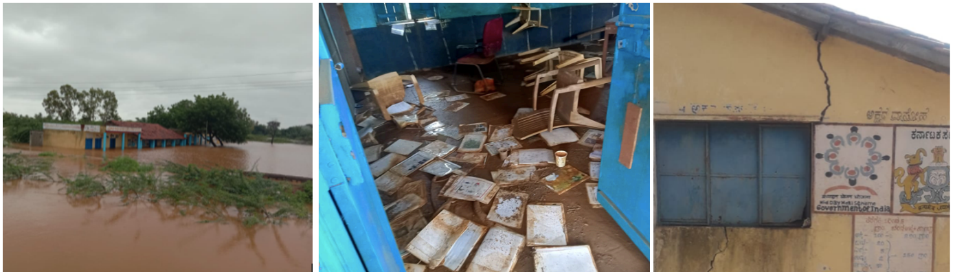
Figure 2: Damages due to floods @ Chikkodi, Karnataka
