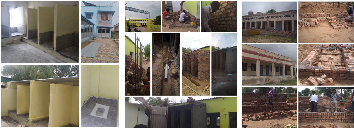
Figure 1: Sewa toilet units under construction @ Sikhar, Rajasthan.
