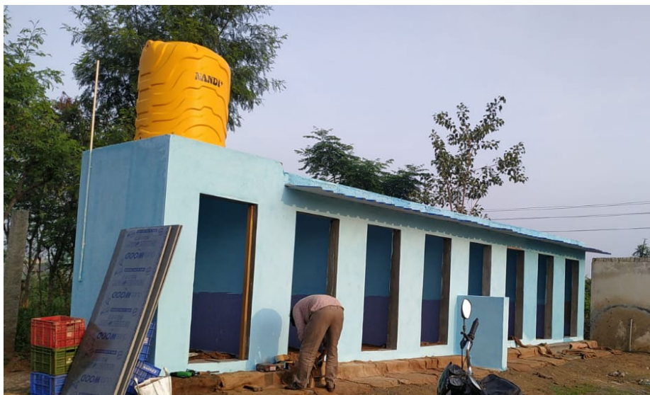
Figure 2: Installed sewa toilets @ Kolar, Karnataka
