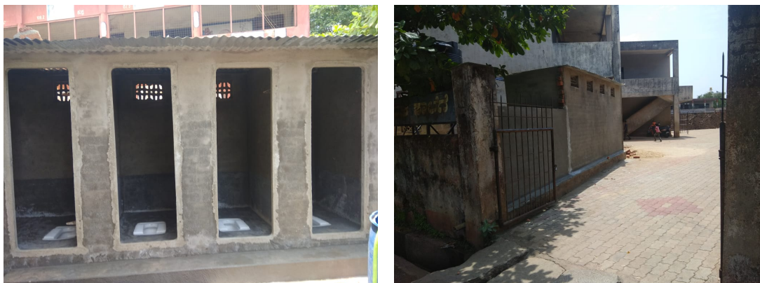
Figure 3: Bio-toilets under construction at Government school no 17, Belagavi, Karnataka
