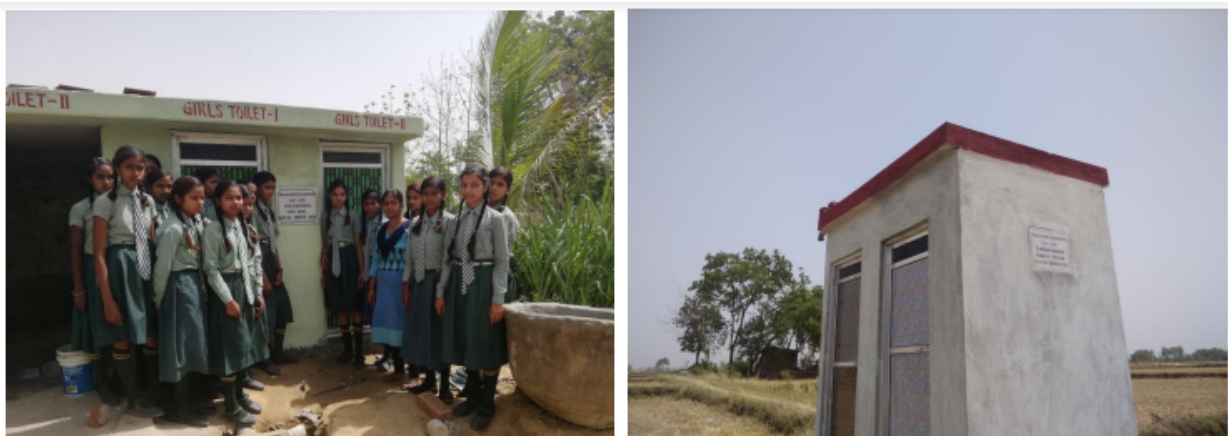
Figure 2: Installed Bio-toilets at Vaishnavi Convent school (left) Ravi Gyan Deep Academy (right) Mirzapur, Uttar Pradesh
