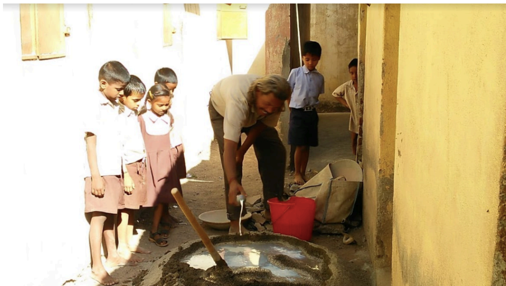
Figure 3: Repair and renovation work at Urdu Primary school, Miraj, Maharashtra.
