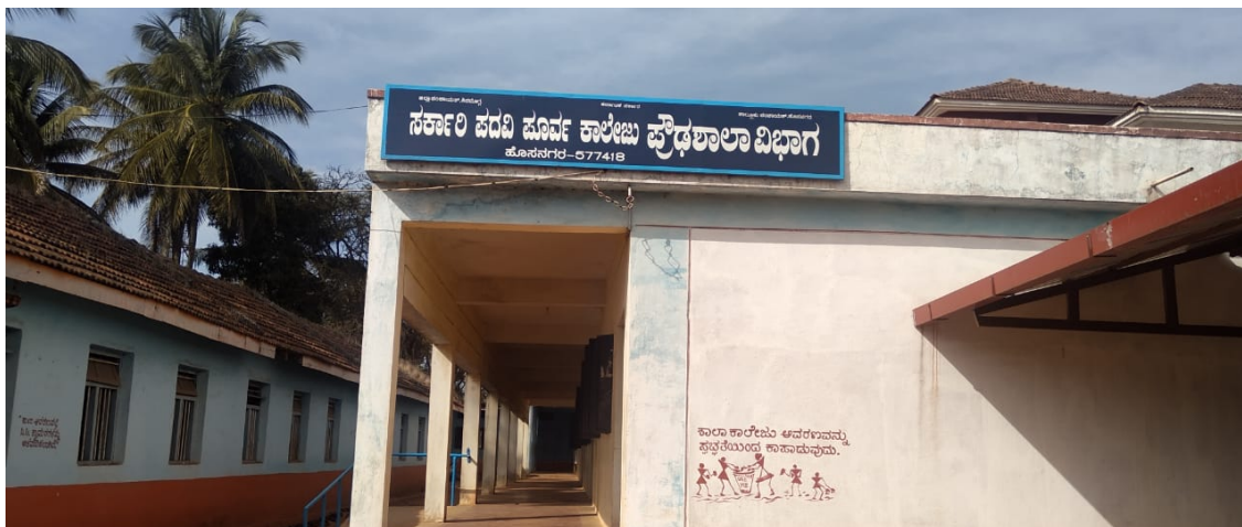
Figure 2: Government high school and college, Hosanagara, Shimoga - Karnataka
