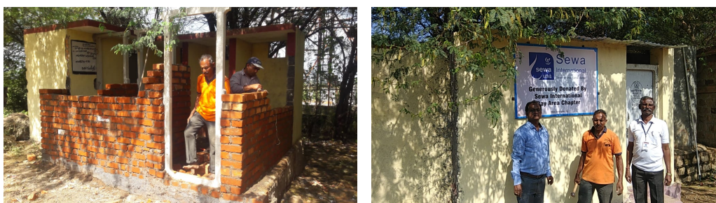
Figure 1: Bio-toilets under construction @ Belgaum, Karnataka
