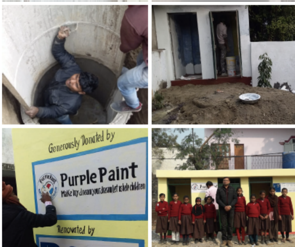
Figure 2: Bio-toilets under construction @ Gorakhpur and Lucknow, Uttar Pradesh
