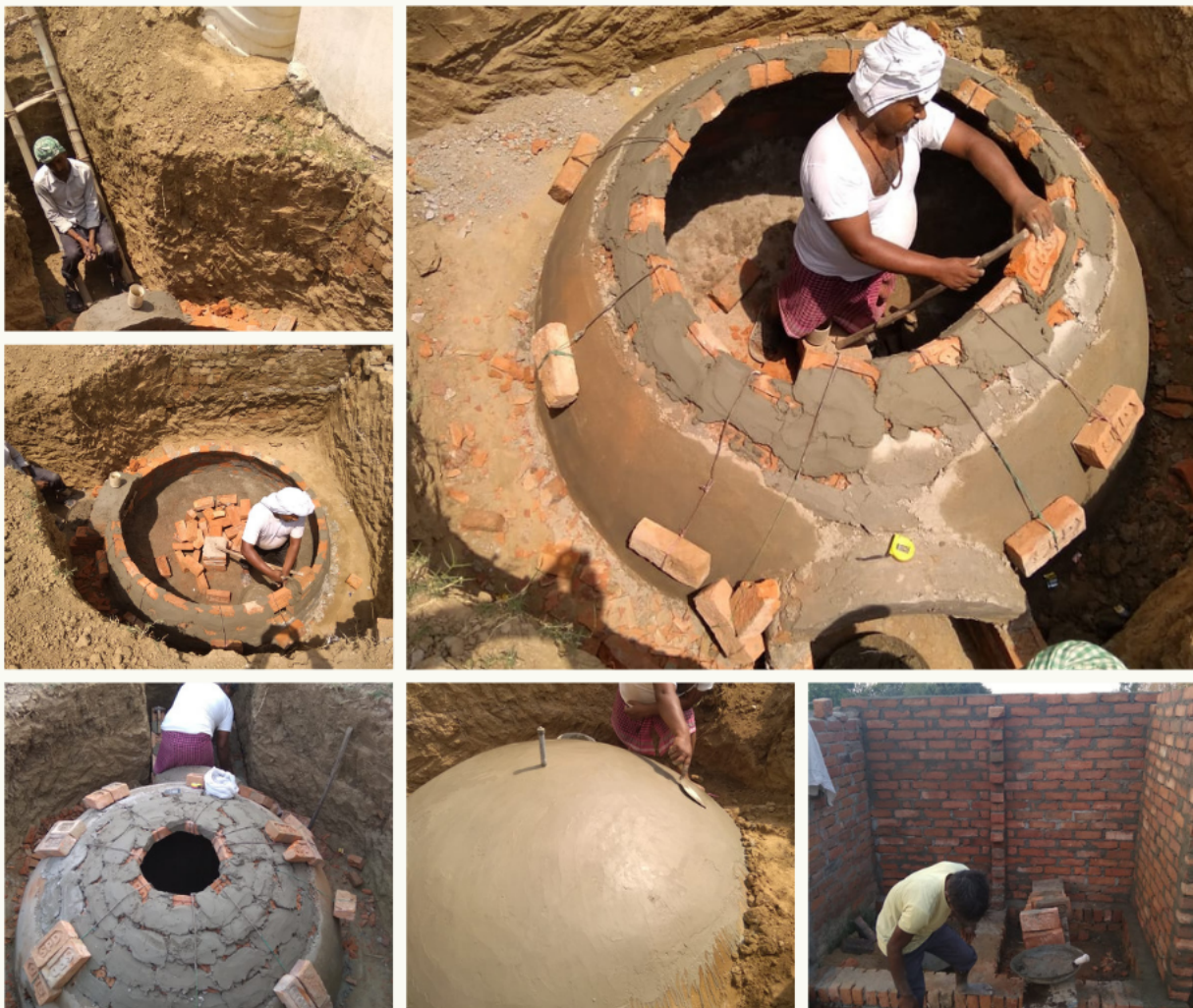
Figure 2: Bio-toilets under construction @ Mirzapur, Uttar Pradesh
