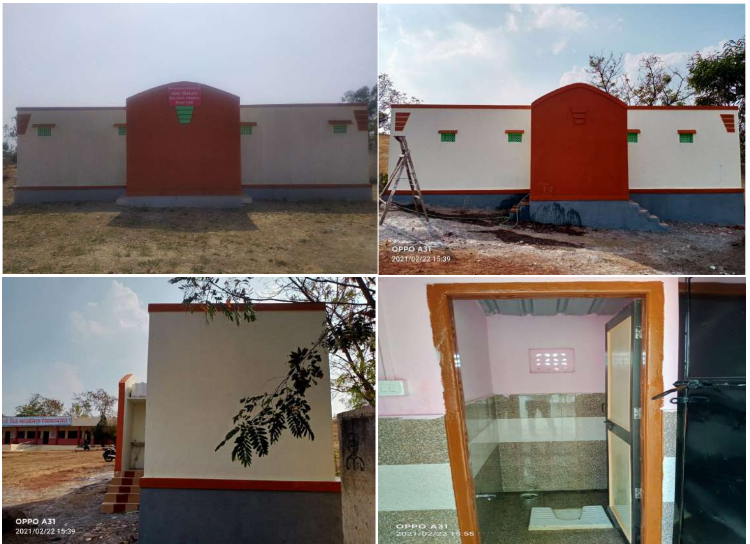
Figure : Toilets constructed at risepise and mahur schools,pune.
