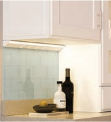
Lighted Power Strip tuned to Warm White (2700K)
