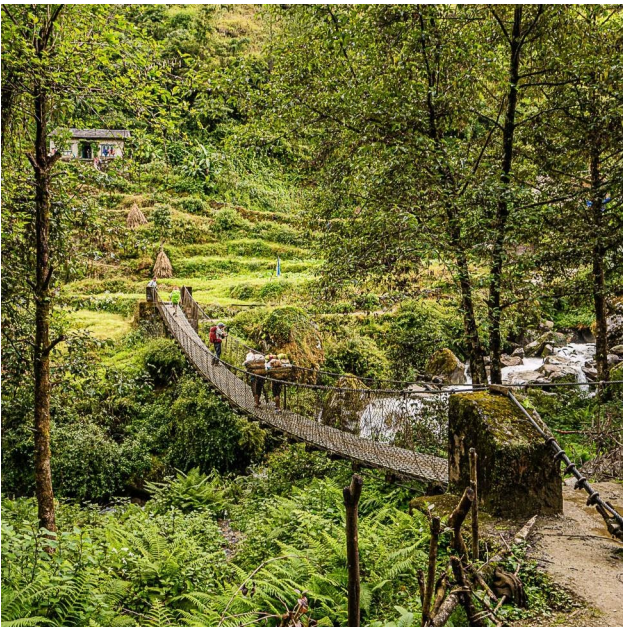
Crossing a suspension bridge on the trail from Phaplu to Lukla
