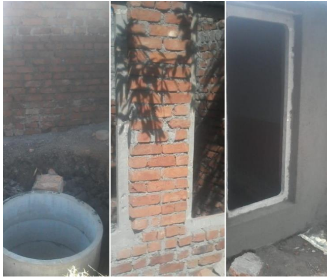
Figure 3: Bio-toilets under construction at Navalgund, Karnataka
