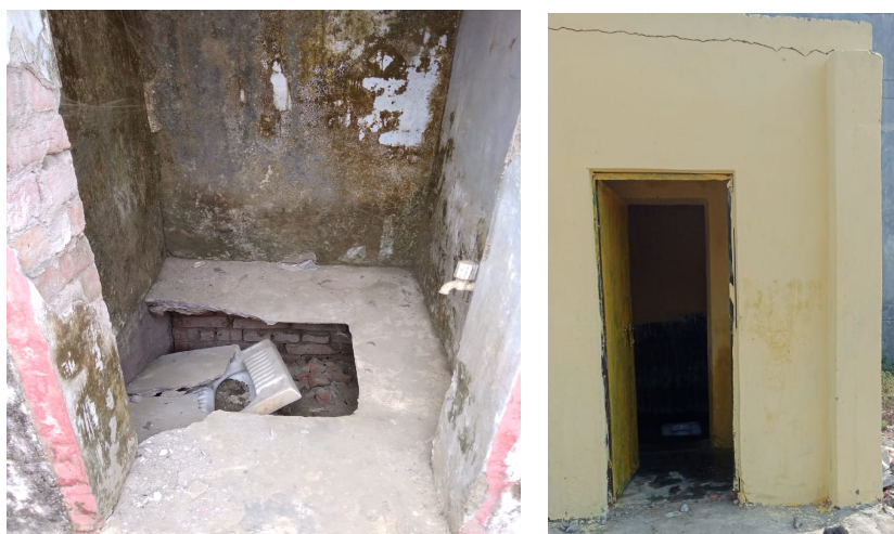
Figure 1: Damaged toilet unit (left), Renovated toilet unit (right) - Primary school Takrohi-2
