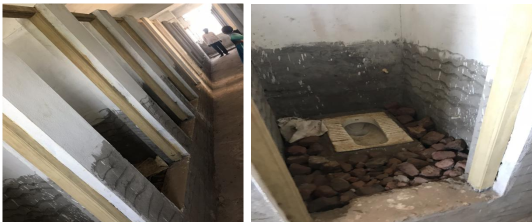
Figure 4: Replaced reinforced concrete cement toilet units - Bidar, Karnataka
