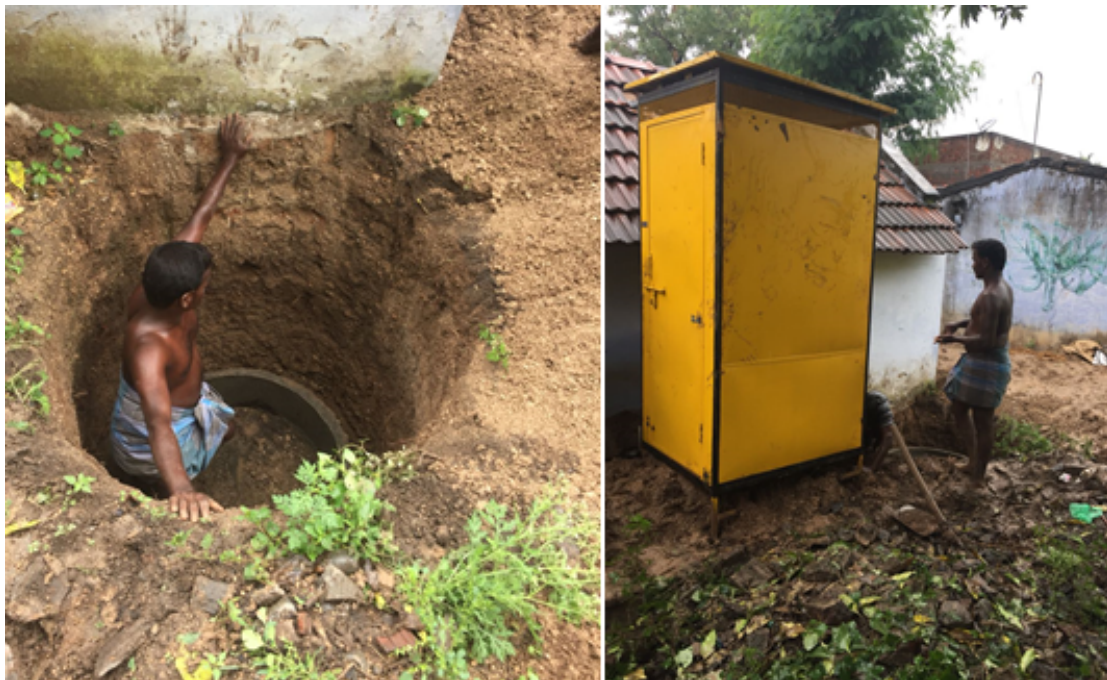
Figure 1: Installation @ Ramayan Patti
