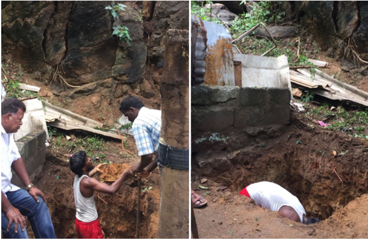
Figure 2: Installation process @ Muthalagu patti, Rockport area
