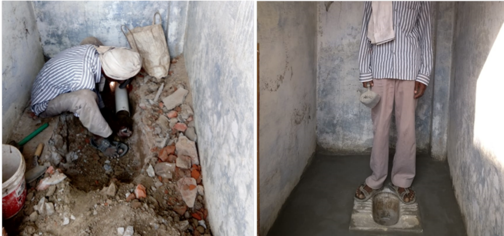
Figure 1: Renovation work at Upper Primary School, Kanosi, Lucknow
