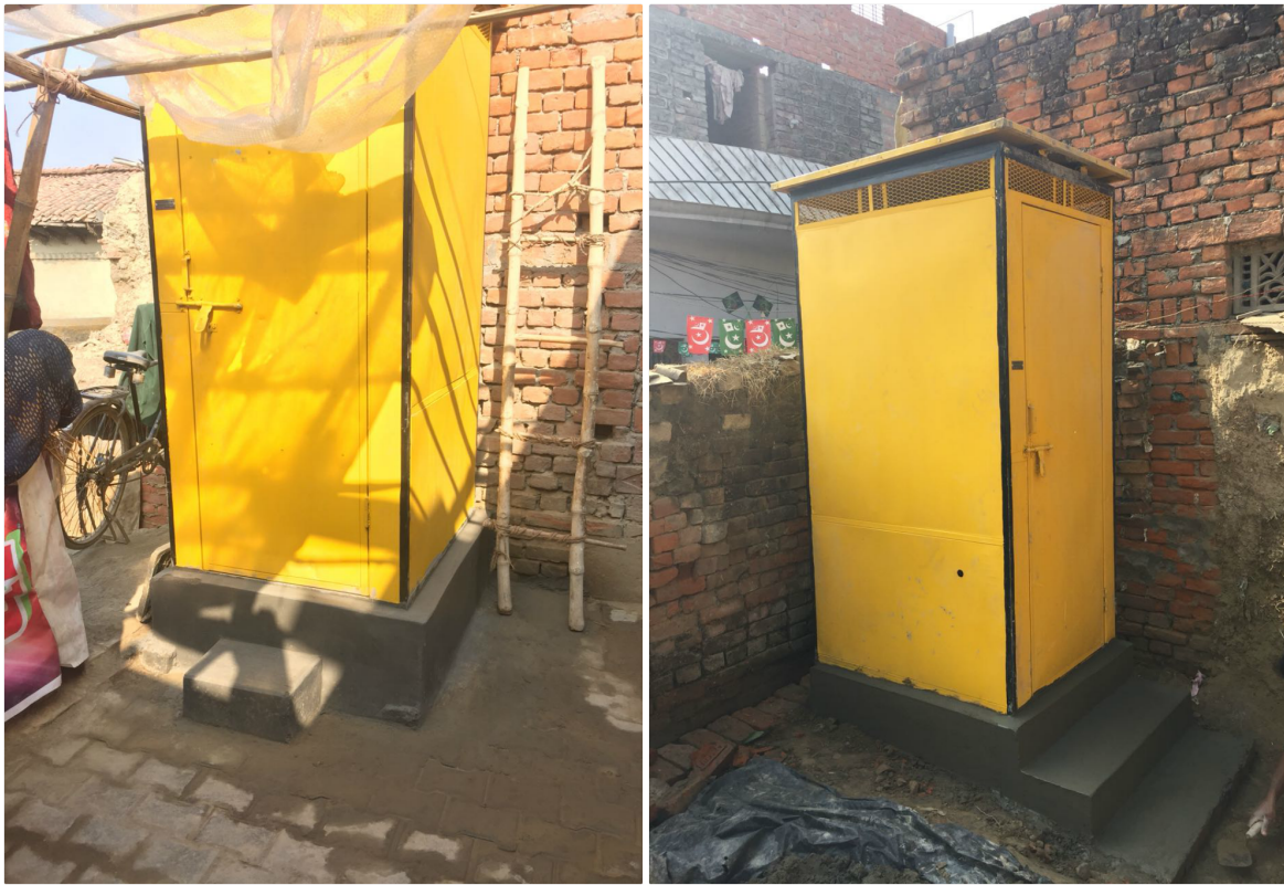
Figure 1: Installed Toilets @ Macharahatta Idga Village, Ramnagar
