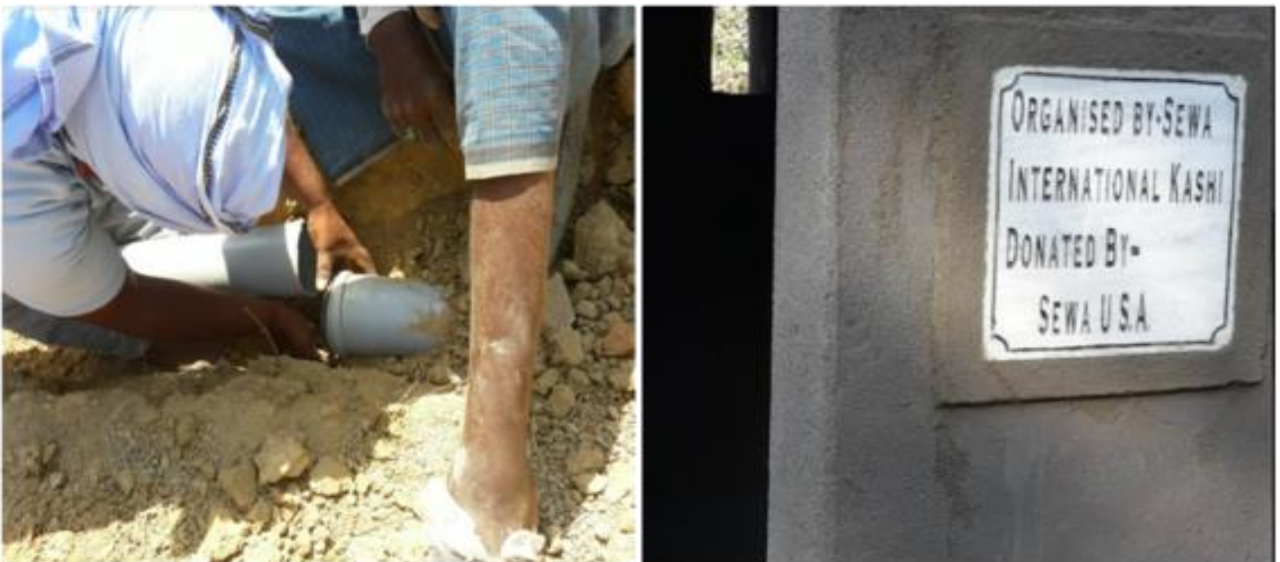
Figure 2: Installation of bio toilet unit @ Chunar
