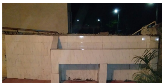
Construction of New wash basin at Hennagara School, Bengaluru
