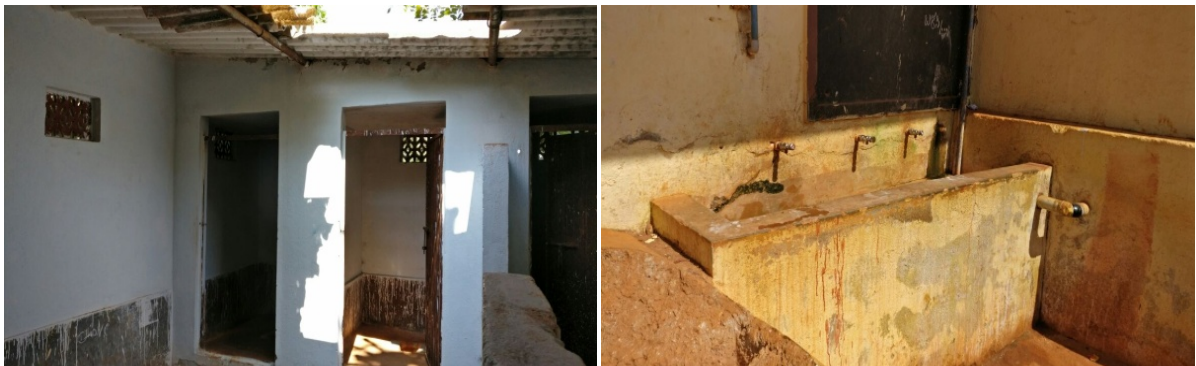
Figure 1: Existing toilet and wash basin at GHPS, Hennagara, Bengaluru.
