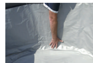
10) Smooth the liner all around the SPA to ensure a good fit.
